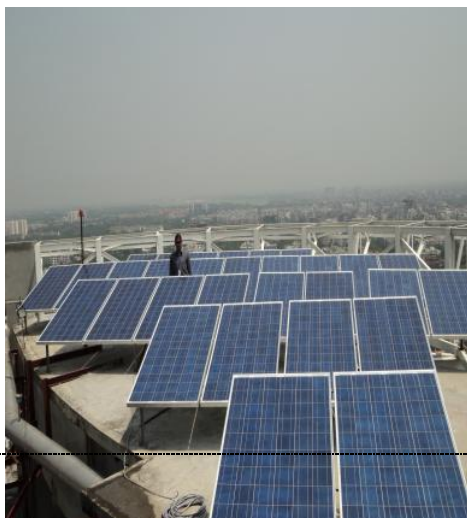
10Kw Solar Power System Installed at Doreen Tower, Gulshan
